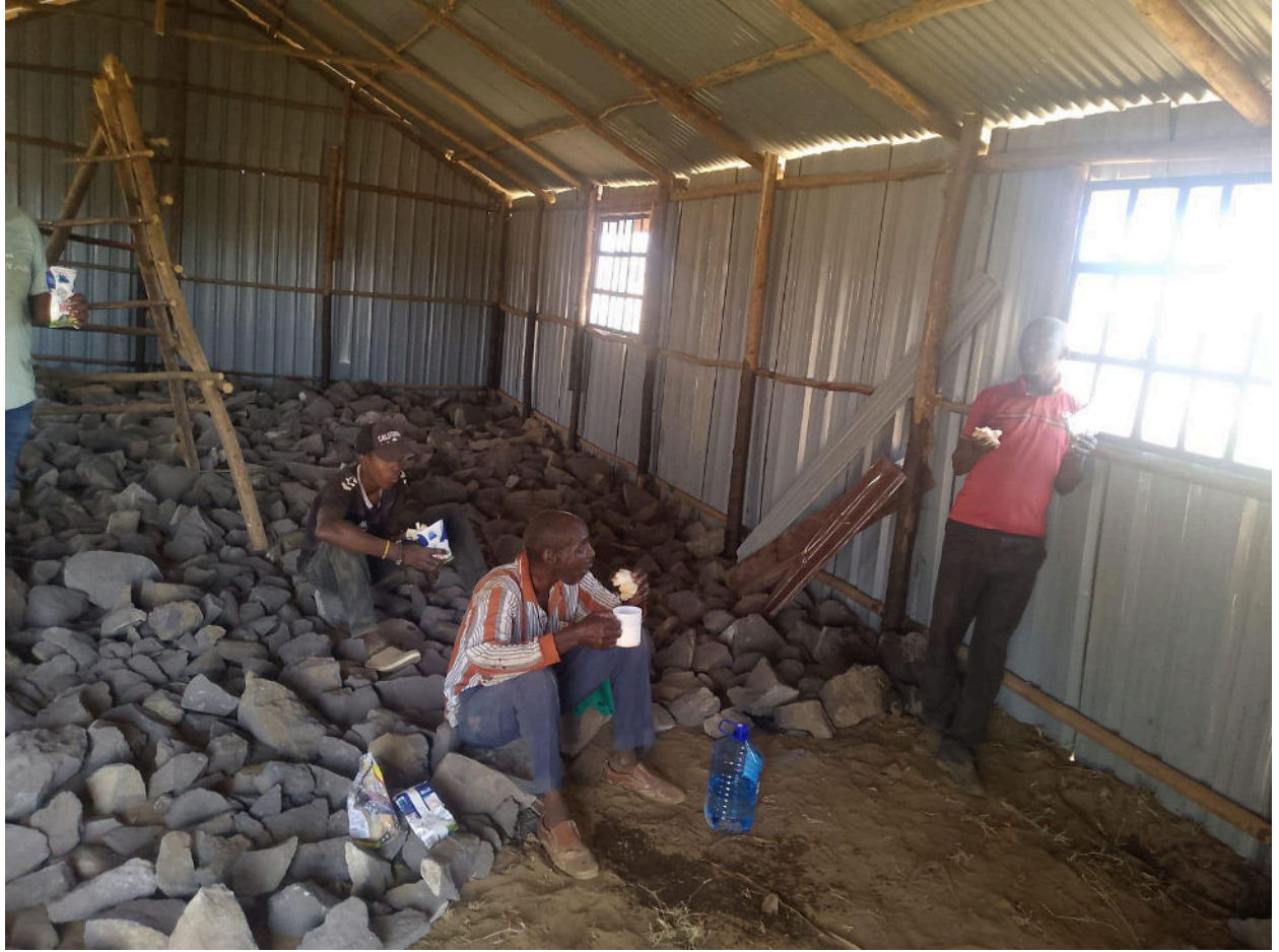
Stage 2: Flooring complete
