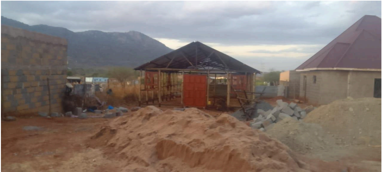
Stage 3: Everything done but flooring and putting glasses on windows
